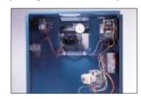
controls instead of a combination control, Burnham has simplified control replacement and reduced replacement costs. The location of the controls also makes regular servicing easier because everything is up front.
