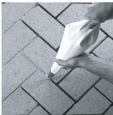
Figure 25 - Grouting Brick
