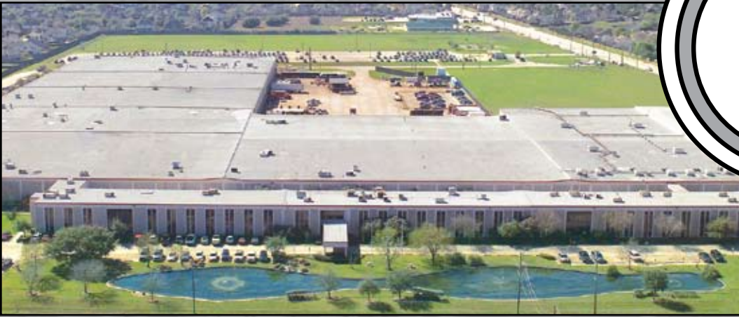
North American Headquarters and Manufacturing Facility (Houston, TX)
