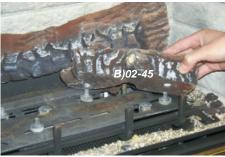
5) Place the Middle Left Log C)02-56 on the two pins as shown.
